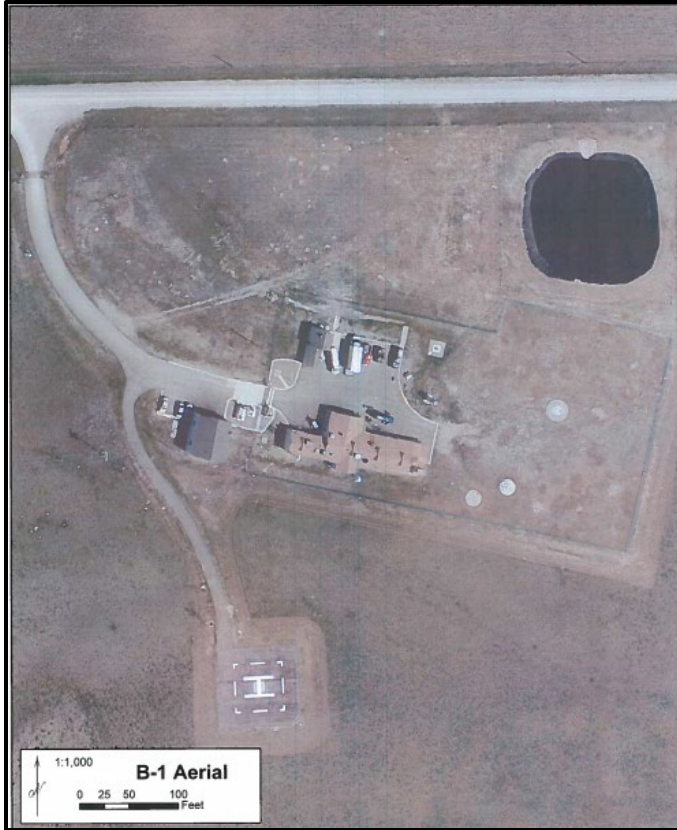
Figure 2: Aerial view of B-01 MAF.
