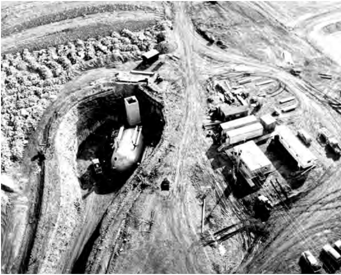
A Launch Control Facility under construction near Malmstrom AFB, Mont. Cold War requirements to build up U.S. nuclear defenses speeded up Minuteman site construction. Builders often labored year-round in three shifts, seven days a week. The Army Corps of Engineers Ballistic Missile Construction Office and its contractors built 1,000 silos between 1961 and 1966. (Image courtesy of the National Museum of the Air Force.)
